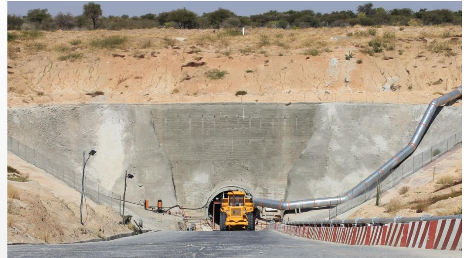
Sand portion of the access decline complete, basalt tunnelling underway
