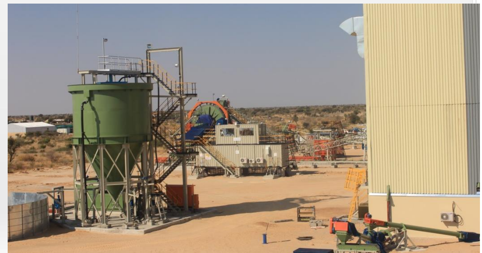
Plant construction complete and awaiting commissioning
